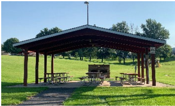
Lower Shelter House – Swimming Pool Park
